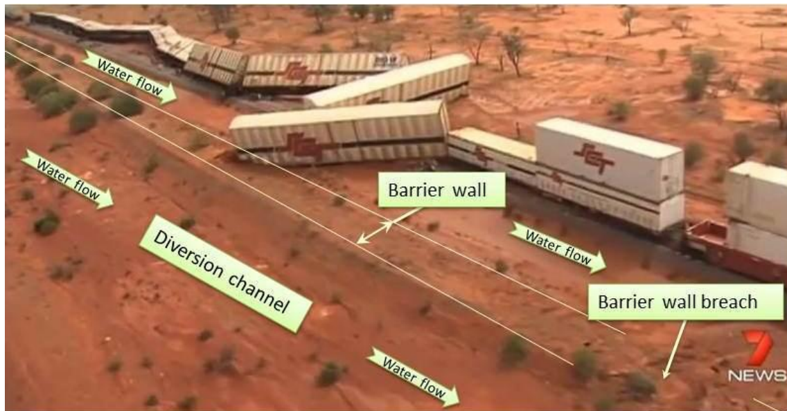
Figure 6: Water diversion channel and barrier wall near the point of derailment
